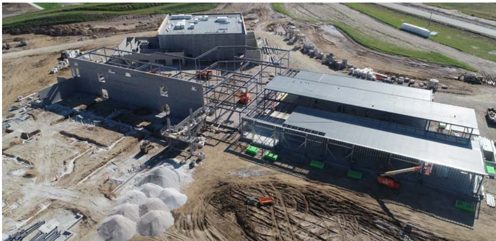
Meadow View Elementary Construction Photo Credit: Mark Miller
